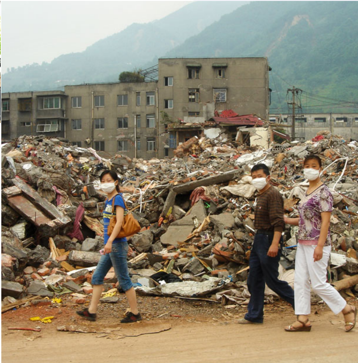
Right: Many school buildings collapsed, while surrounding buildings did not. In the mountain villages, Caritas Germany is rebuilding kindergartens, schools and a residential home for the elderly.
