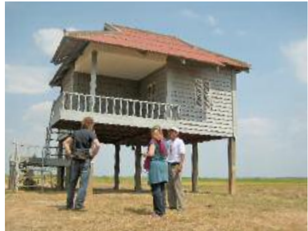
Traditional construction methods with improved protective functions. Stilt houses have already protected many people against inundations in South and Southeast Asia.
